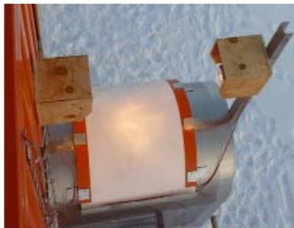
Installation of a wooden shield to prevent radiation from the external IR lamps to disturb astronomical measurements
