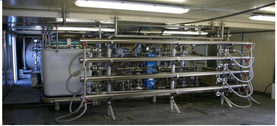
Desalination sea water plant reverse osmosis system (Max capacity of 28.000 lts/day)
