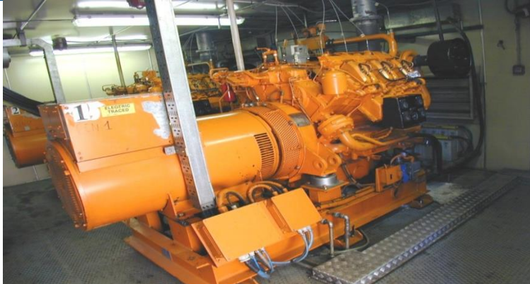
Combined heat power system (500 MWh/Y)
