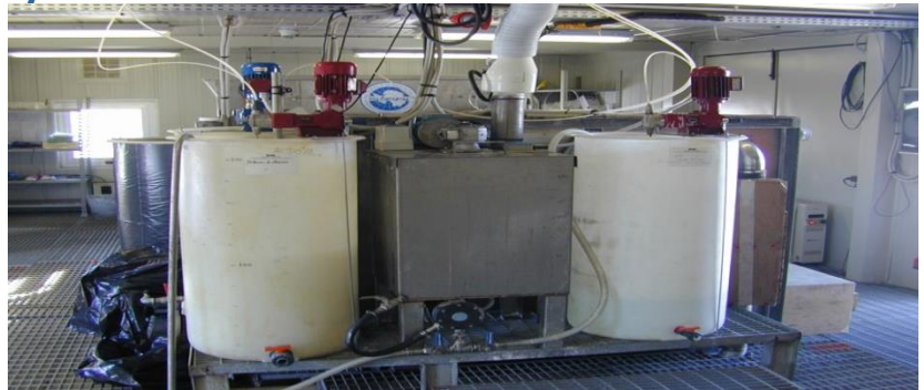
Desalination sea water plant reverse osmosis system (Max capacity of 28.000 lts/day)
