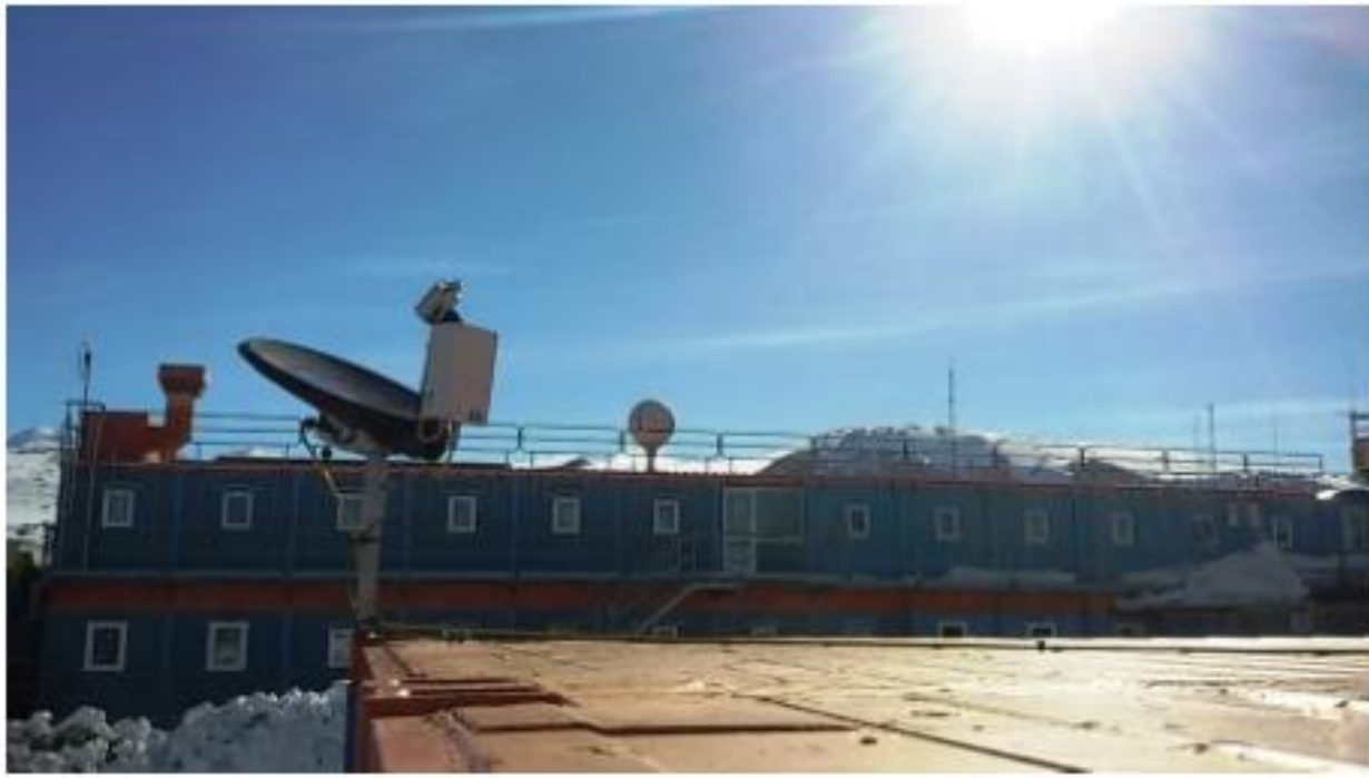
Micro Rain Radar at Mario Zucchelli research station on the roof of the logistic container.
